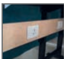
In built Sockets
